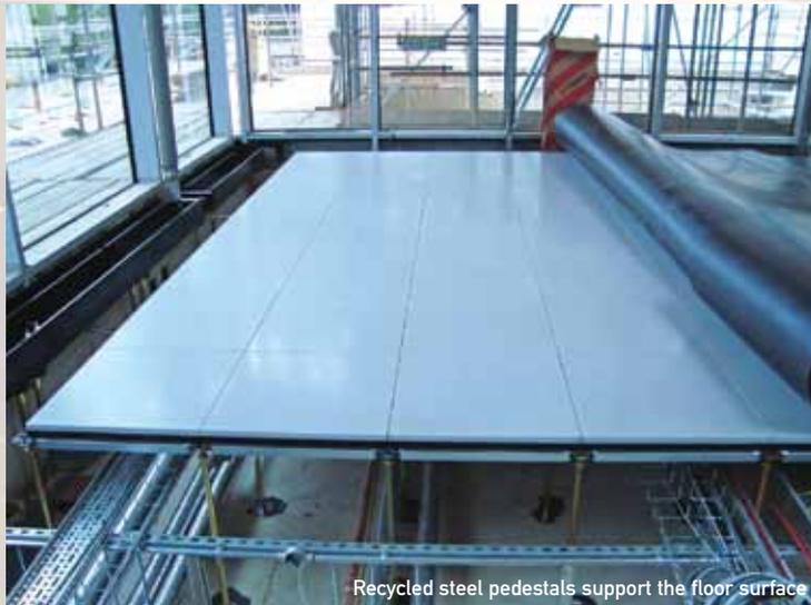
Recycled steel pedestals support the floor surface
